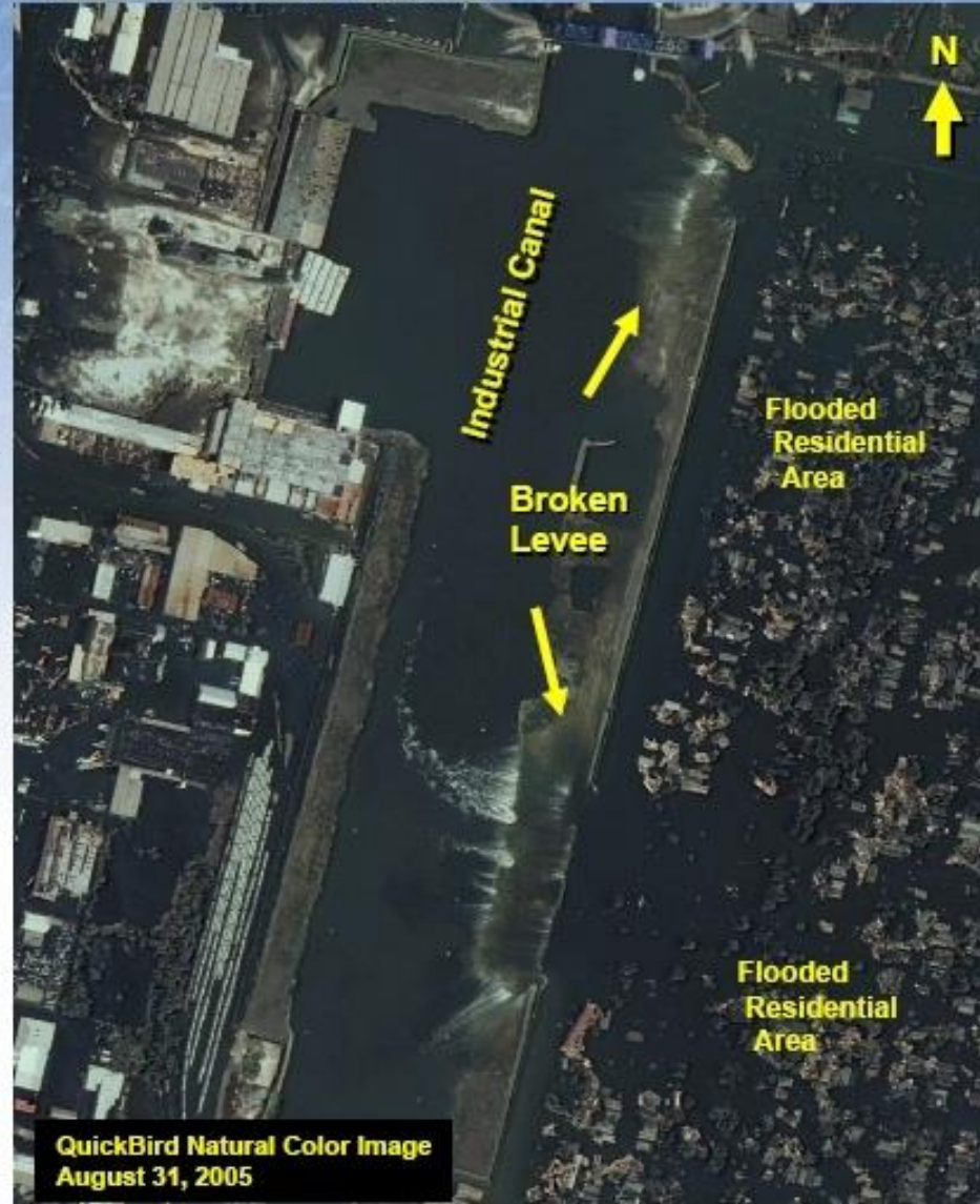
After Hurricane Katrina
